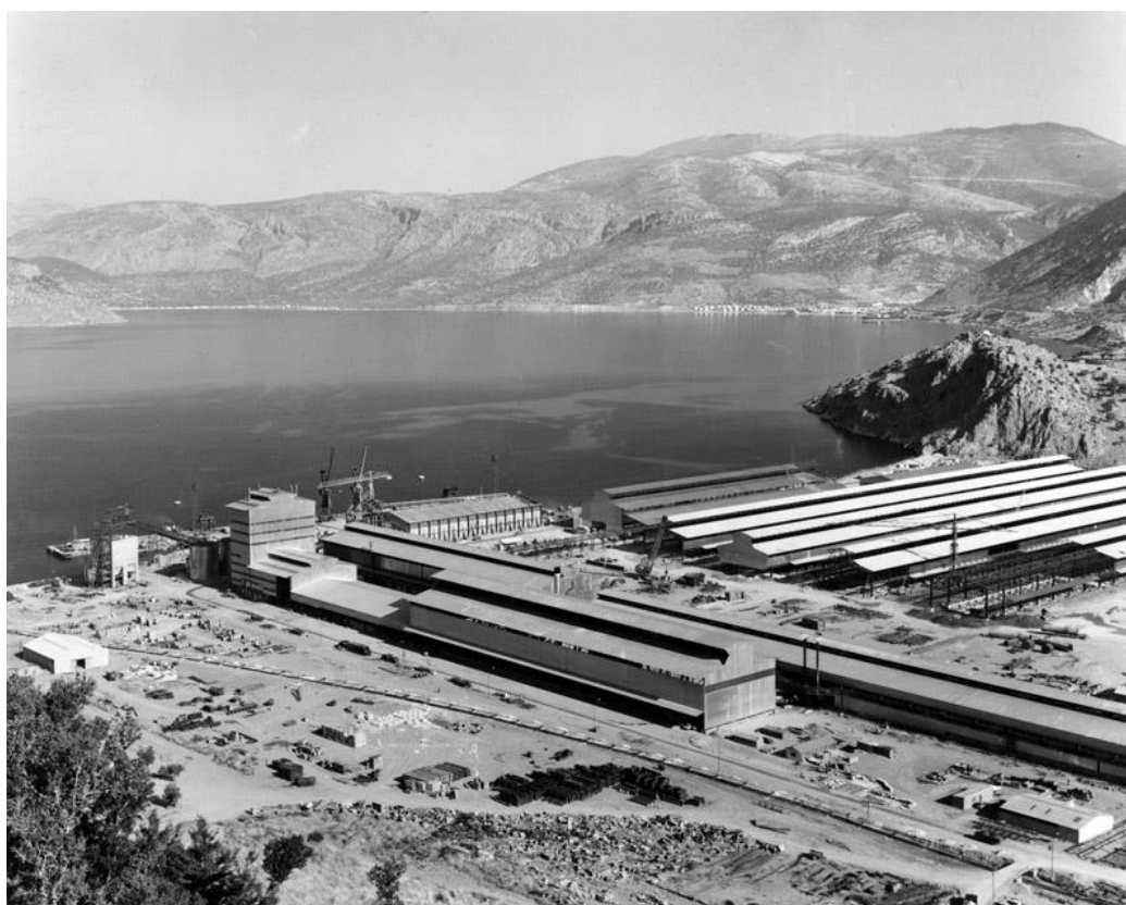
Figure 2. Aluminium of Greece, Saint-Nicolas plant, general view (1963-1966). © Photographic collection of Aluminium Français.
